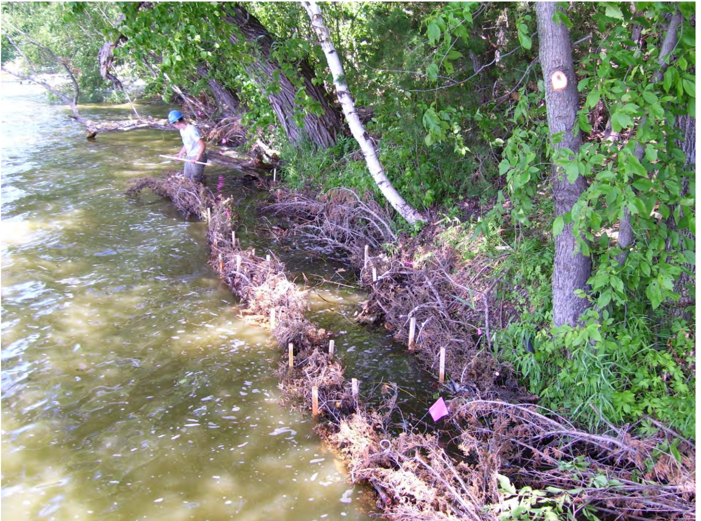
Brush Bundles being installed with 4 foot hardwood stakes
