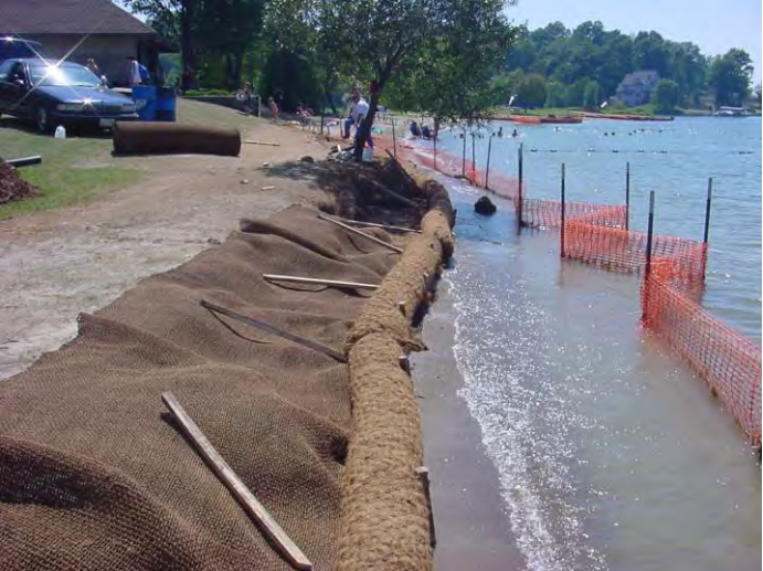
Installing coconut-fibre rolls
