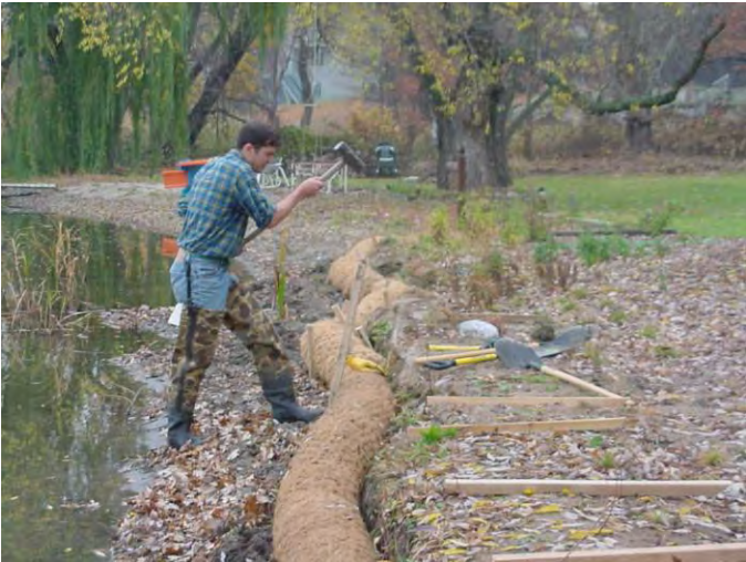
Installing coconut-fibre rolls
