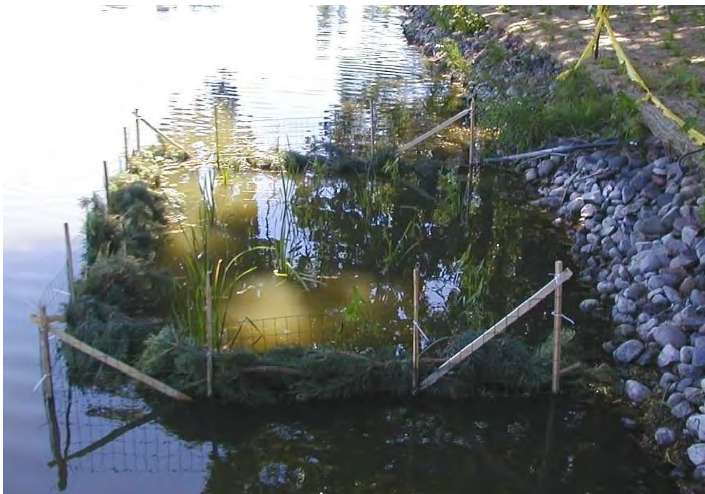
Godlewski, Rush Lake 2008. In this example the pine trees have been compressed by bundling them with cord. This method creates a denser and more effective wave breaker. A 2 foot wire fence has been installed on the outside to exclude muskrats from the planting.
