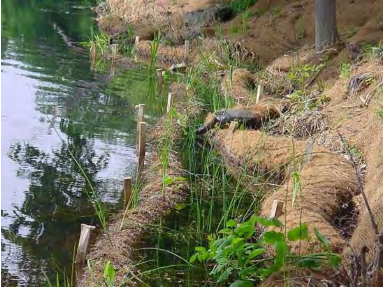
Coconut-fiber rolls installed
